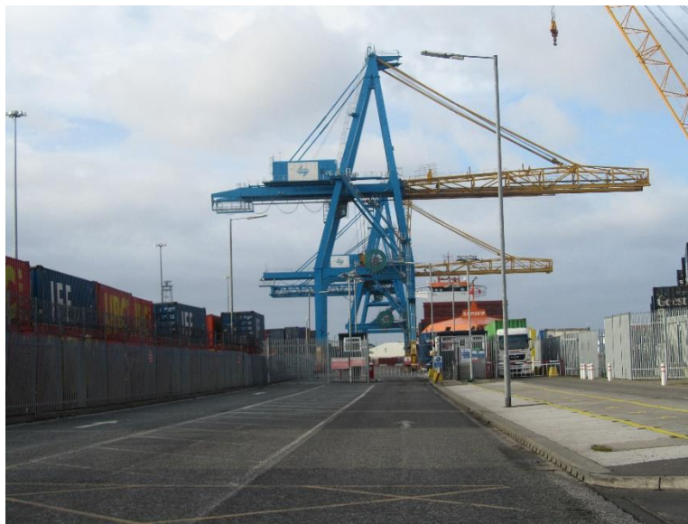
Figure 6: Fixed Guideway Crane. Source: Author.
