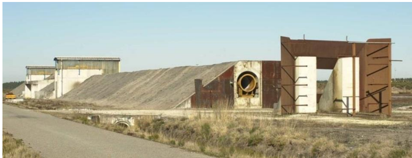
Figure 1. External view of the facility showing the cannon muzzle and the blow deflectors
