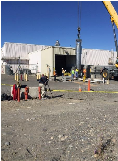
Figure 6. Horizontal Unloading of NAC-LWT at PNNL
