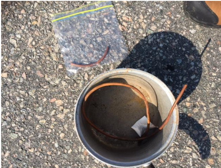
Contaminated cable found in the North Bay event
