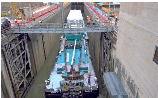
Fig. 10. Passing the lock of Lauffen/Neckar.
