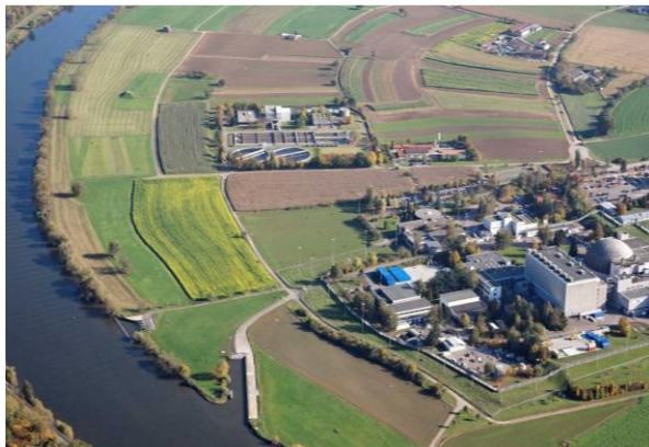
Fig. 2. Nuclear Power Plant Obrigheim including berth with RORO ramp.
