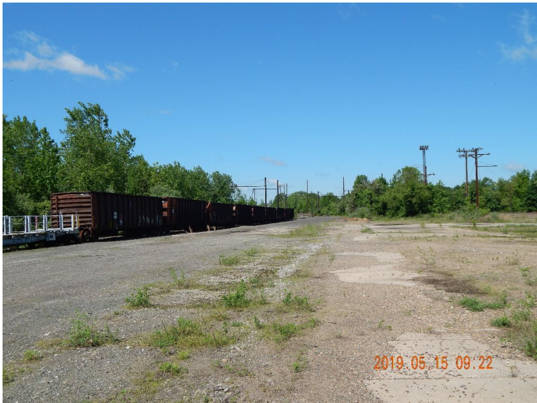
Figure 8 Spur at Morrisville Railyard looking west
