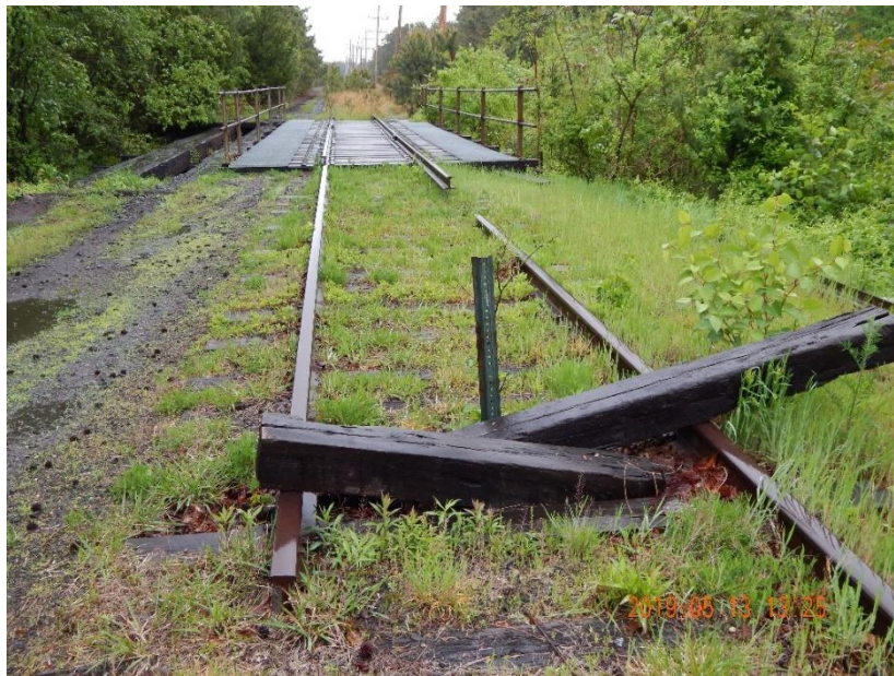
Figure 5 Rail at Lakehurst New Jersey looking northeast
