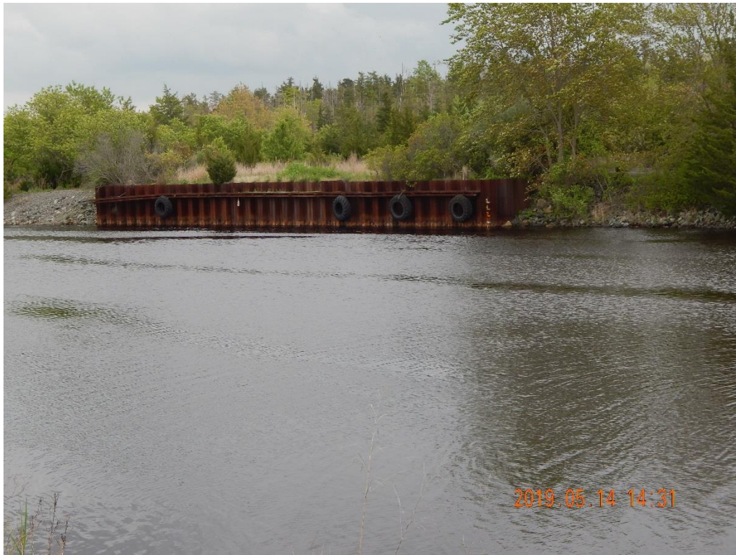
Figure 12 Oyster Creek barge access (south bank of Oyster Creek)
