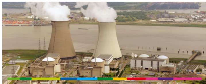
Figure 6 Doel Nuclear Power Plant
