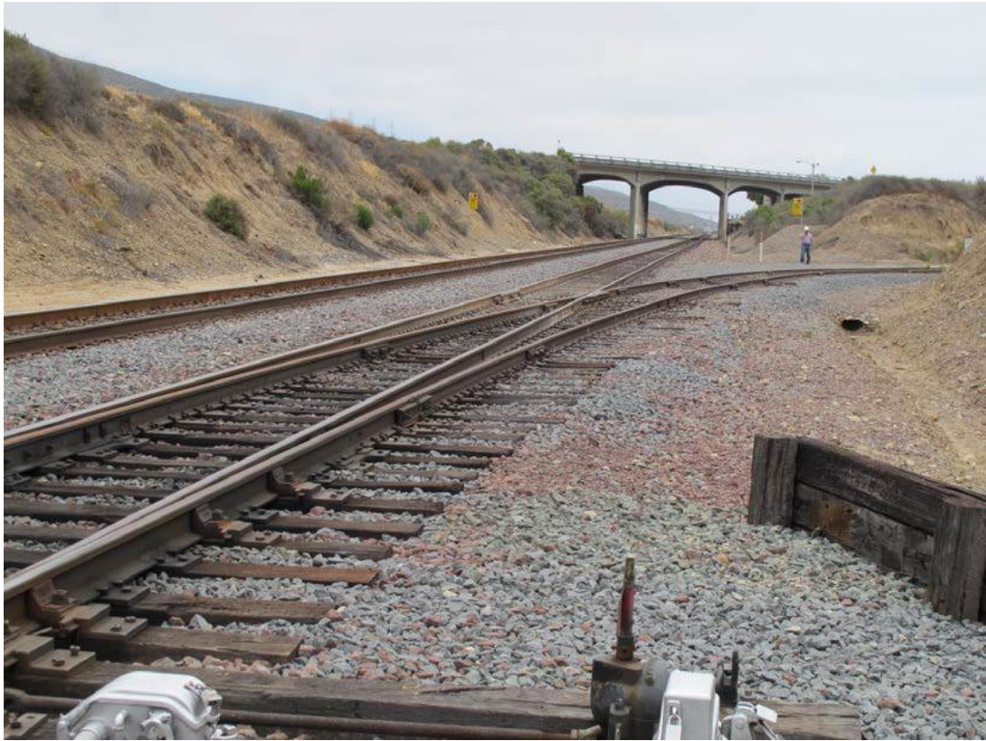
Figure 9 Junction of on-site rail spur and mainline at San Onofre (2015)
