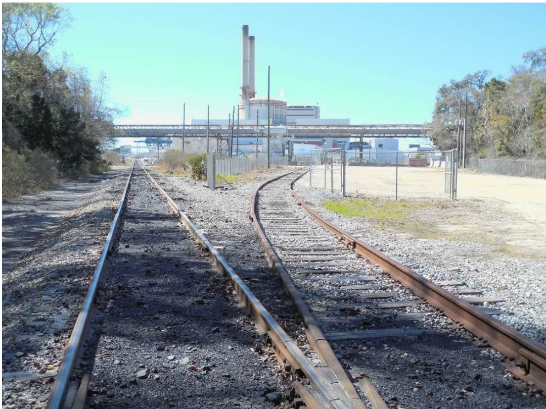
Figure 10 On-site rail spur at Crystal River (2015)
