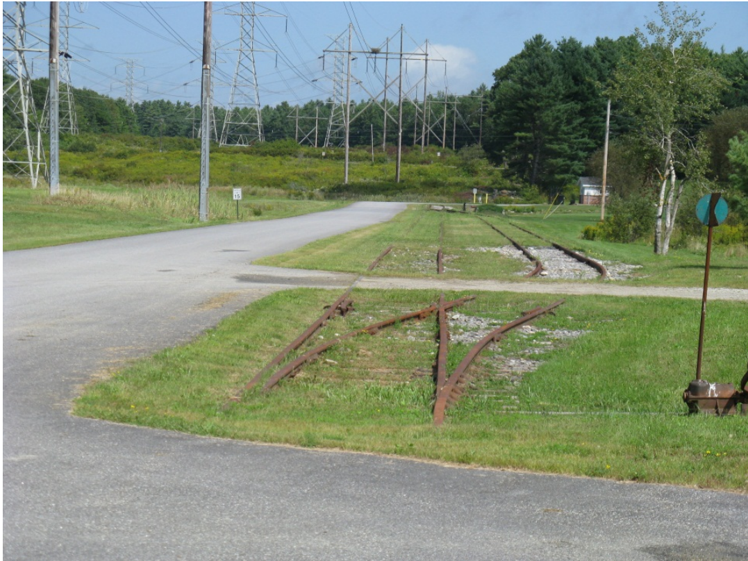
Figure 5 Condition of onsite rail system at Maine Yankee (2012)
