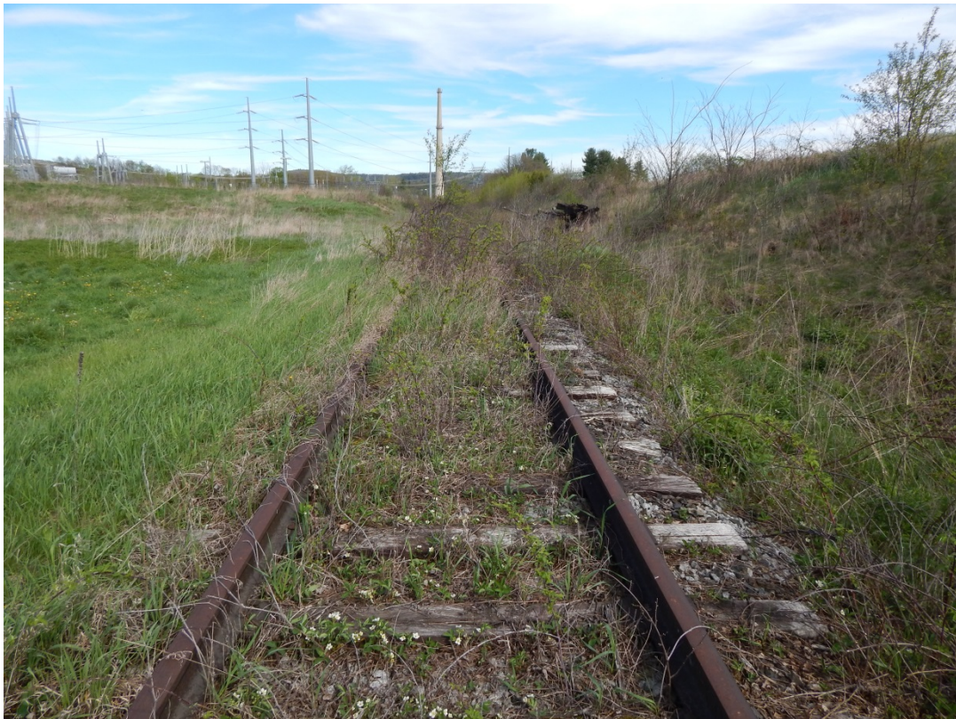
Figure 6 Rail spur approaching Vermont Yankee site entrance (2016)
