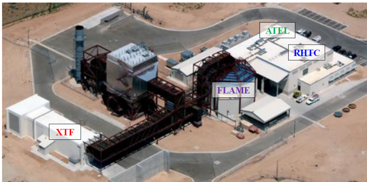
Figure 1. A large quiescent burn room (FLAME), a cross-wind burn tunnel (XTF), a radiant heat fire simulator (RHTC), and a high temperature thermal environment lab (ATEL), comprise the Thermal Test Complex.
