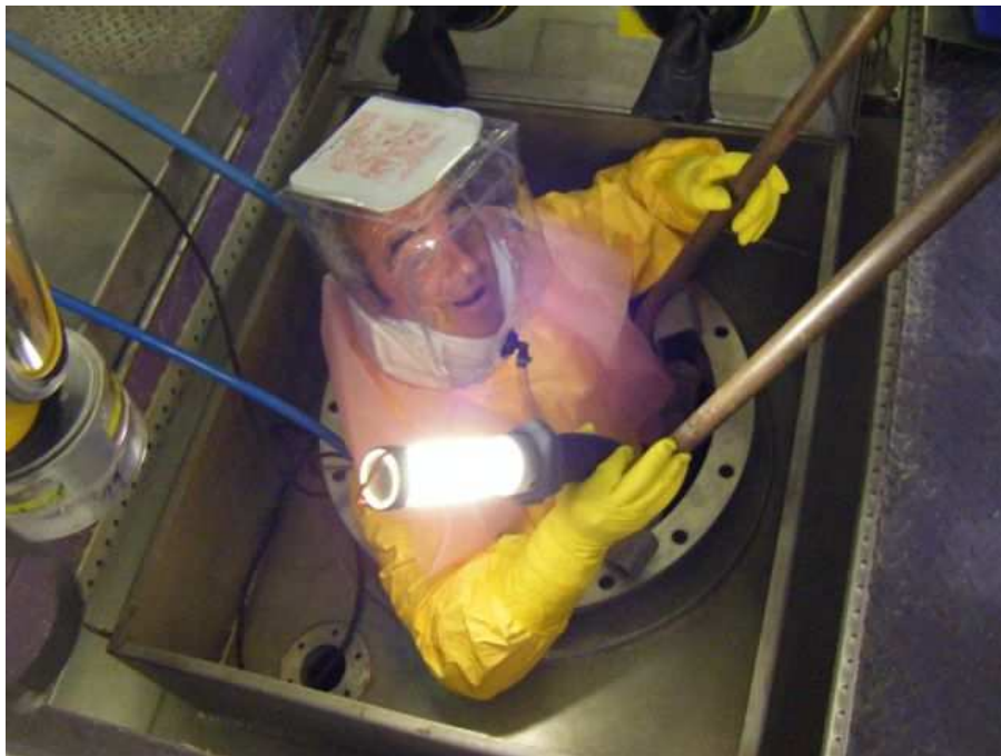
Figure 4. Operator in ventilated protective clothing entering the cavity
