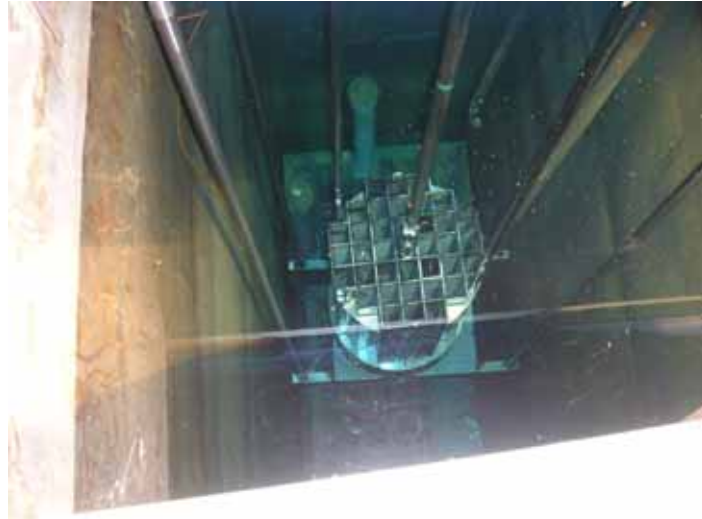
Figure 8. Loading SNF inside the pool into the basket
