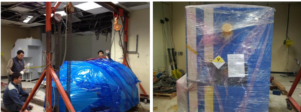
Figure 4. Dismantling by special working group and preparation for transportation
