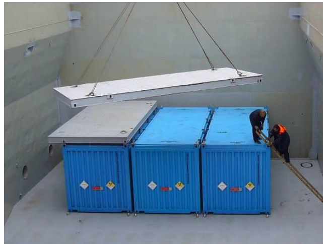
Fig. 11. Loading the ISO containers with the SKODA VPVR/M casks inside into the hold of the MCL-Trader vessel
