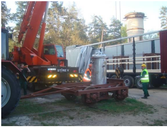
Fig. 1. Installing the TUK-19 casks onto a truck (a) and into a TK-5 rail car (b)
