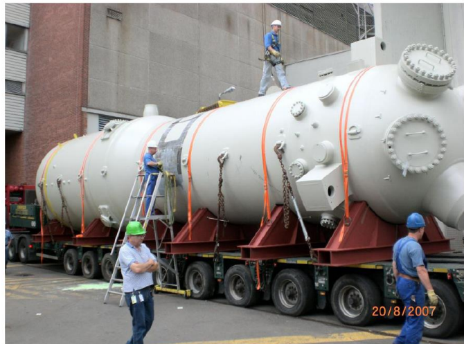
Fig. 2 Transport of Spent Steam Generator [4]
