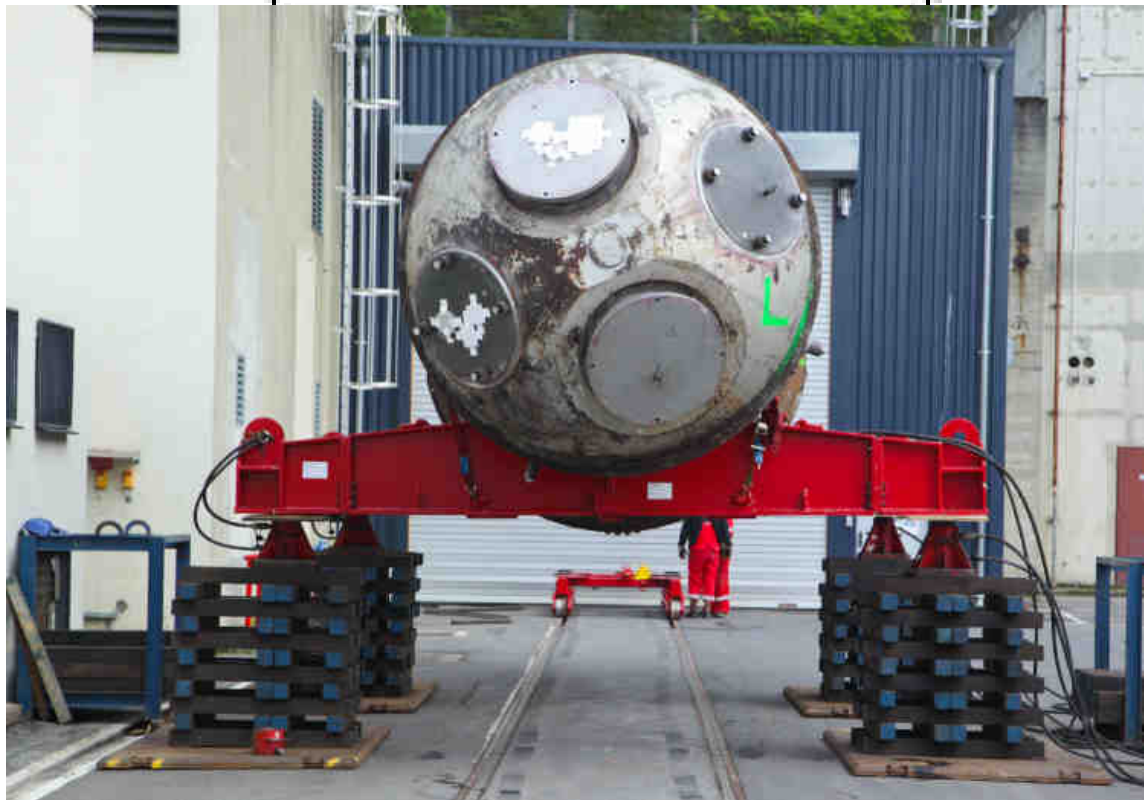
Figure 9. The SG was lifted by a jacking system
