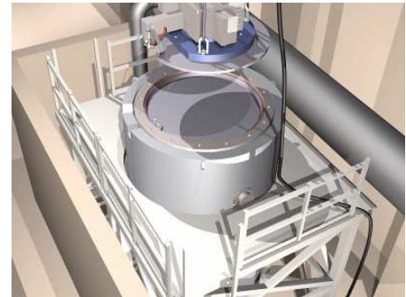
Figure 10, Placing Lid on RWC
