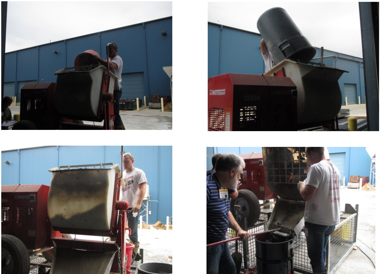
Figure 14. Mixing and pouring Packcrete.
