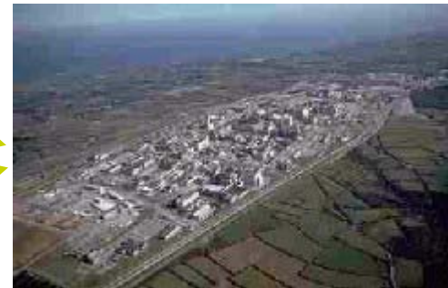
AREVA La Hague reprocessing plant
