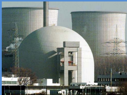
Nuclear Power Plant BIBLIS (GERMANY)
