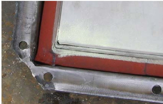
Figure 4 An IP-2 post drop testing showing the migration of test dust across the seal boundary during a transient leak
