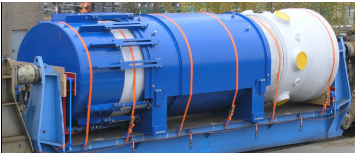
Figure 1. Reactor pressure vessel (white) including additional shielding elements and transport frame (blue) - NPP Rheinsberg (Picture: EWN)
