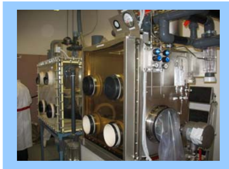
Pu transfer in to shielded GB
