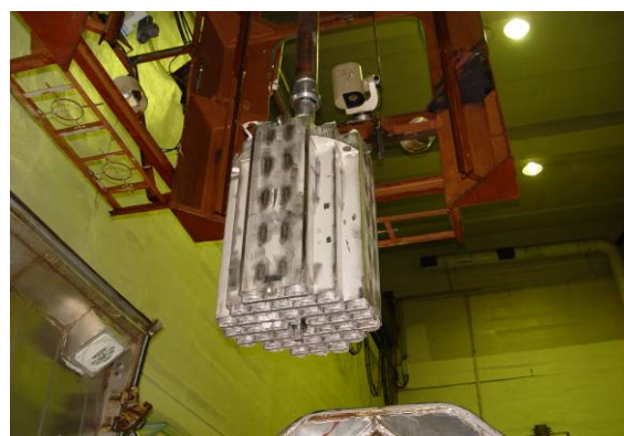
Figure 4. Basket being lifted out of the cask using the central suspension/hanger.
