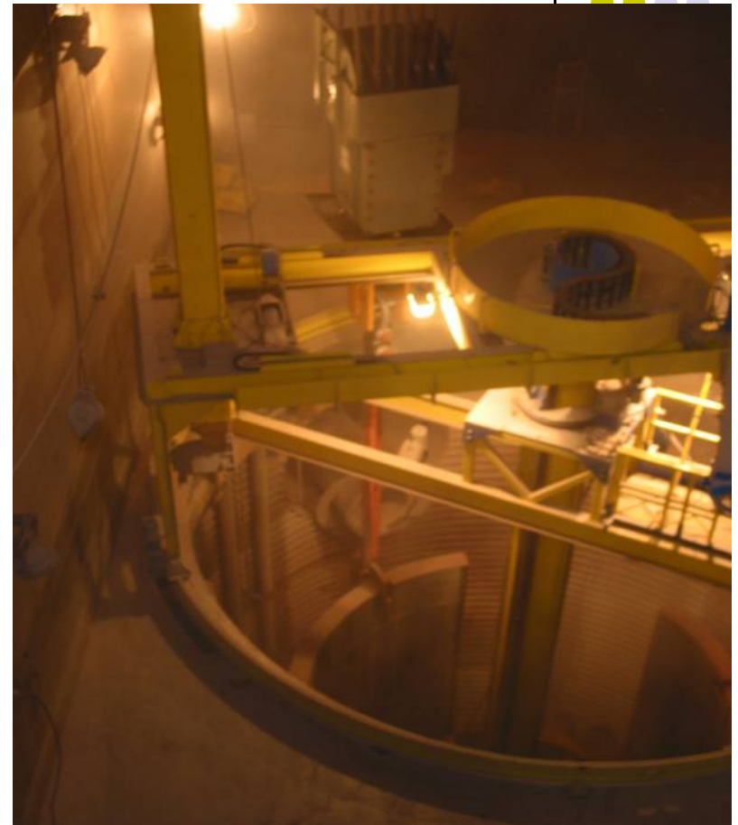
Rigging and removing a beltline section from the vessel
