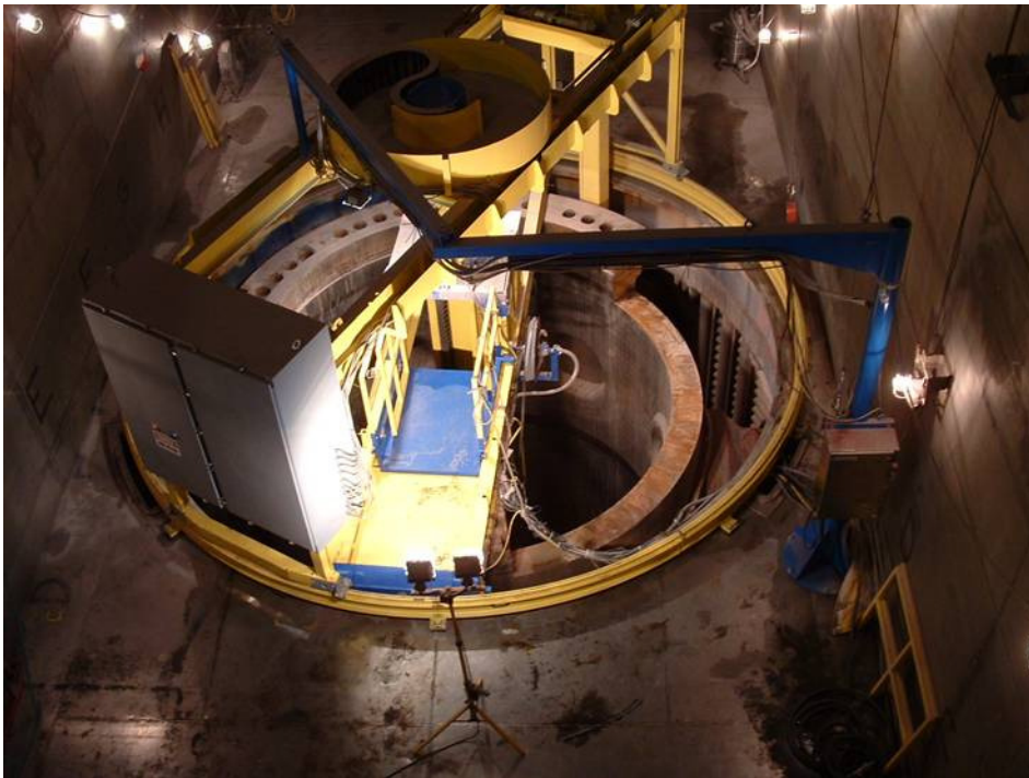
Segmenting a section of Vessel Flange
