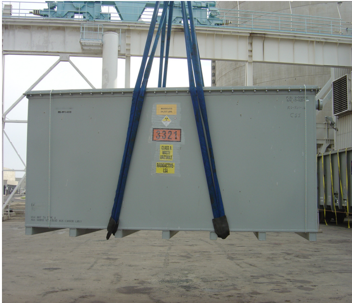
Type A Box with Core Support Shield Sections
