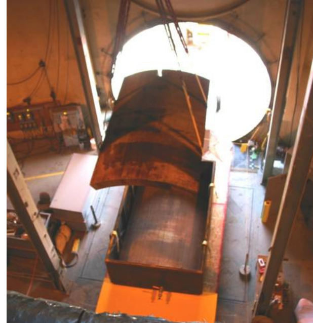
Beltline section packaged into metal box prior to introduction of grout
