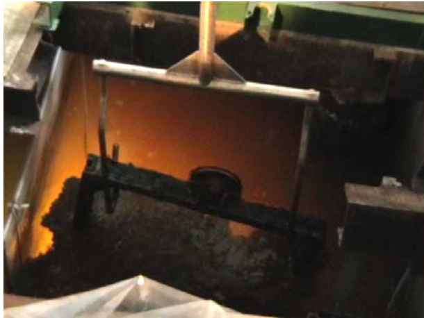
Figure 5. Vinča spent fuel basin, carbon steel removal operations
