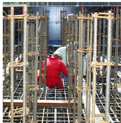
Fig. 1. Construction of the unyielding target realized by a reinforced concrete block with the dimension of 14 m x 14 m x 5 m depth and a mass of 2,450,000 kg.
