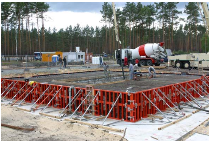
Fig. 1. Construction of the unyielding target realized by a reinforced concrete block with the dimension of 14 m x 14 m x 5 m depth and a mass of 2,450,000 kg.
