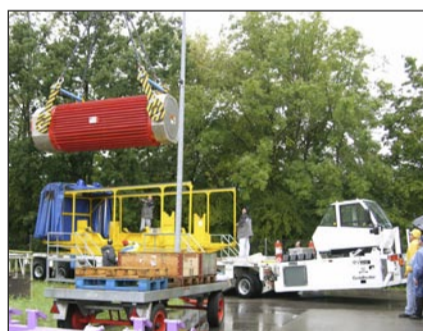
The transport to the Swiss Central Interim Storage Facility ZWILAG in August 2004 was performed by using a mobile crane (400t capacity) and the ZWILAG special truck
