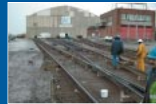
Rail spur under construction
