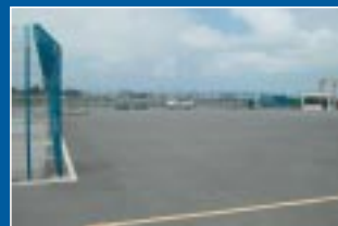
Lorry Parking Facility
