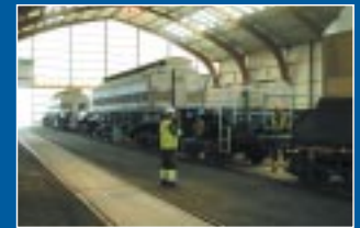
Wagon Parking Facility
