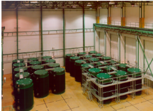
Fig. 2 CASTOR ® 440/84 Casks loaded and stored at Dukovany NPP, Czech Republic
