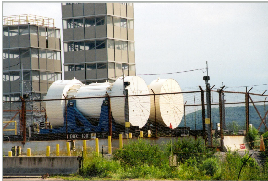
Figure 4. Photograph of the loaded West Valley casks stored within the West Valley Demonstration Project Site.
