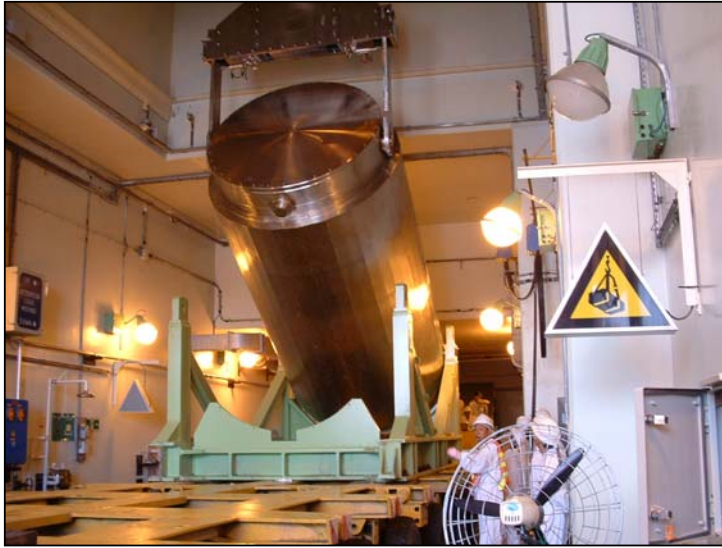
Photo 2 - Upending the STC in Receiving Hall of the KX Building
