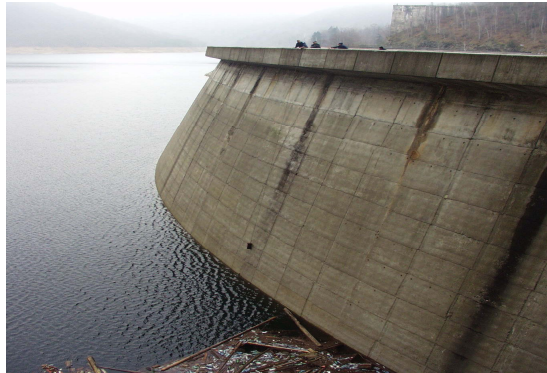
Figure 10 the performing of the immersion test at VIDRARU DAM Lake
