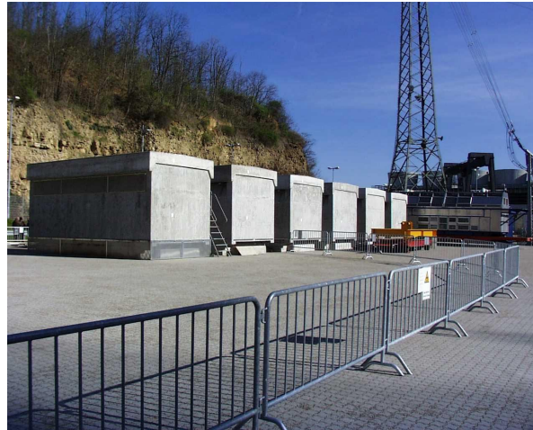
Figure 4, Six Concrete Garages for Storage of CASTOR ® V/19 Casks at Neckarwestheim NPP
