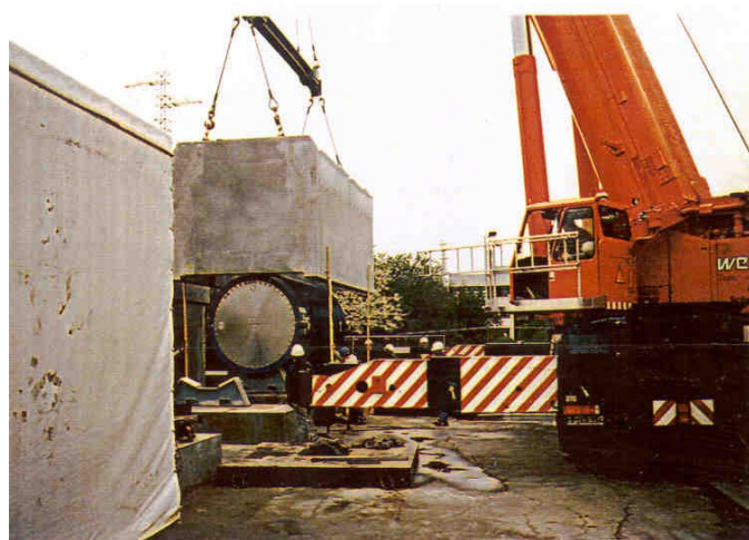
Figure 5, Concrete Garages for Storage of CASTOR ® V/19 Casks at Biblis NPP
