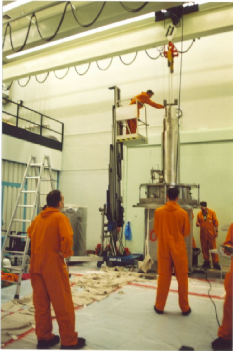
Transfer of TRIGA fuel into the „GNS 16“ at DKFZ Heidelberg
