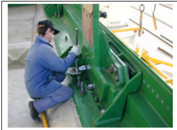
Fig. 7: making up trunnion metal supports with interface parts
