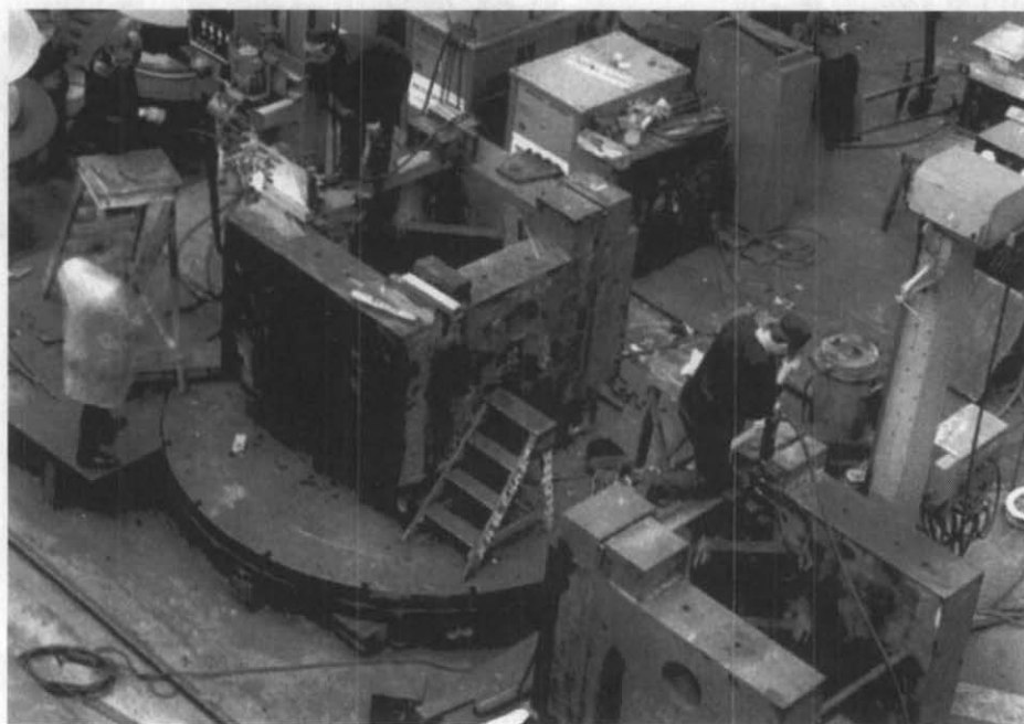
Fig 2 Early Electro Slag Welding
