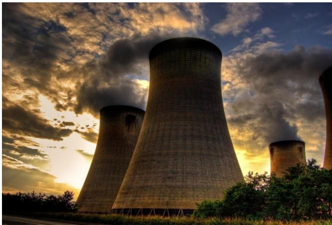
**Figure 1.** Sample hyperboloid cooling tower from the Drax coal-fired power station in the United Kingdom. This image is a reminder that not all cooling towers are nuclear cooling towers, and it reinforces the importance of location information for operational status assessment. Image credit: Jonathan Brennan, via Flickr. Image number 3635530311, 6/12/2009.
