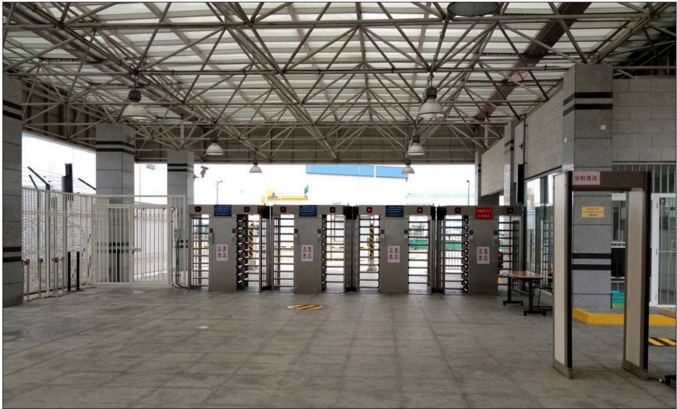
Figure 2. An entrance access to a protected area at Daya Bay nuclear power plant. The floor-to-ceiling turnstile doors and the gate with detector are shown in the photo. Credit: Photo provided by a security expert at the plant, January 2013.
