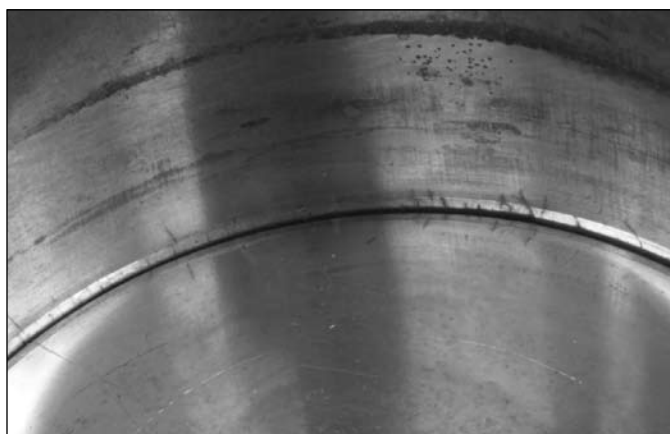
Figure 8. 3013 inner-container welded-top section after exposure to boiling magnesium chloride showing container interior with sidewall and plug cracks
