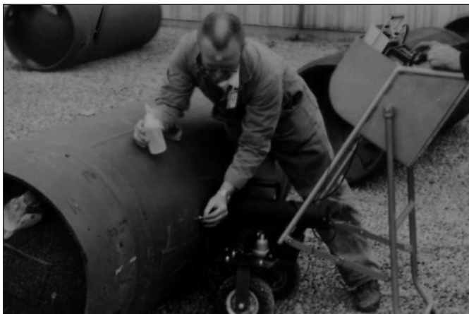
Figure 5. Gamma-ray enrichment measurement by Roddy Walton at the K-25 plant at Oak Ridge in 1969
