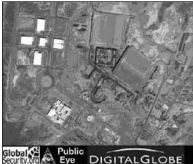
Figure 12: Satellite image of the partially covered enrichment facilities in Natanz (Iran)
