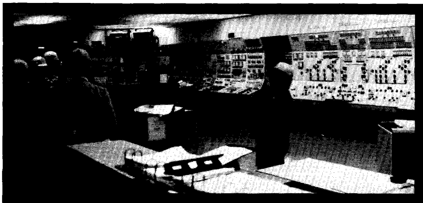
Control room at the Pickering plant.
