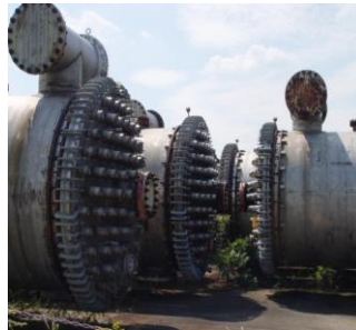
Figure 4 - Heat exchanger lay down
