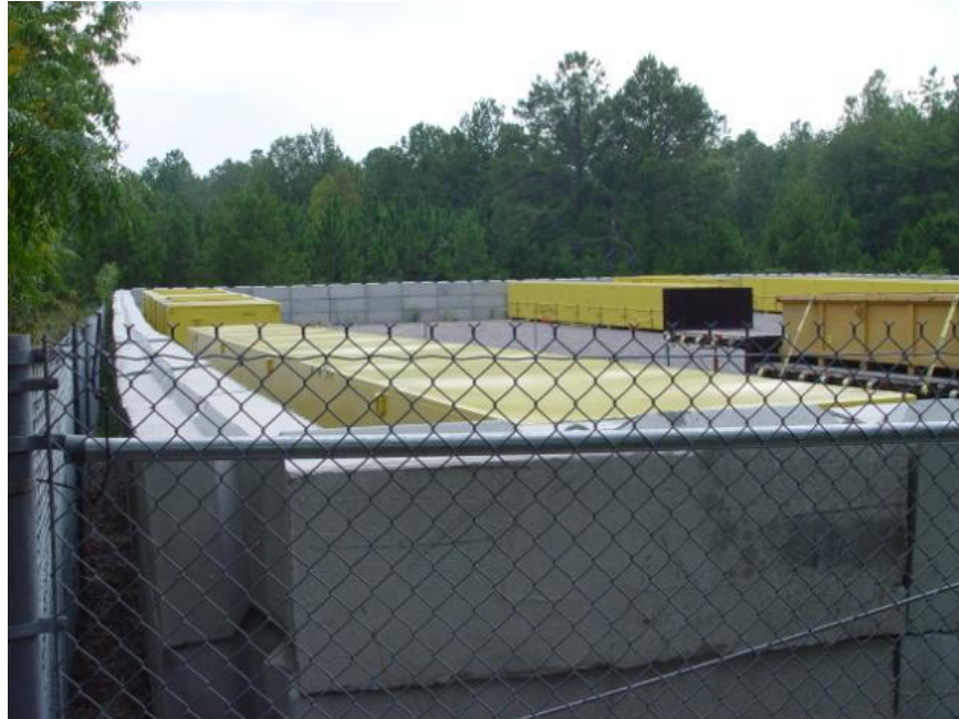
Figure 6 - Shielded Sealand container compound
