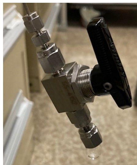
Figure 3. Water bubble forming on at the exhaust of the vessel during drying at 220°C [9].
