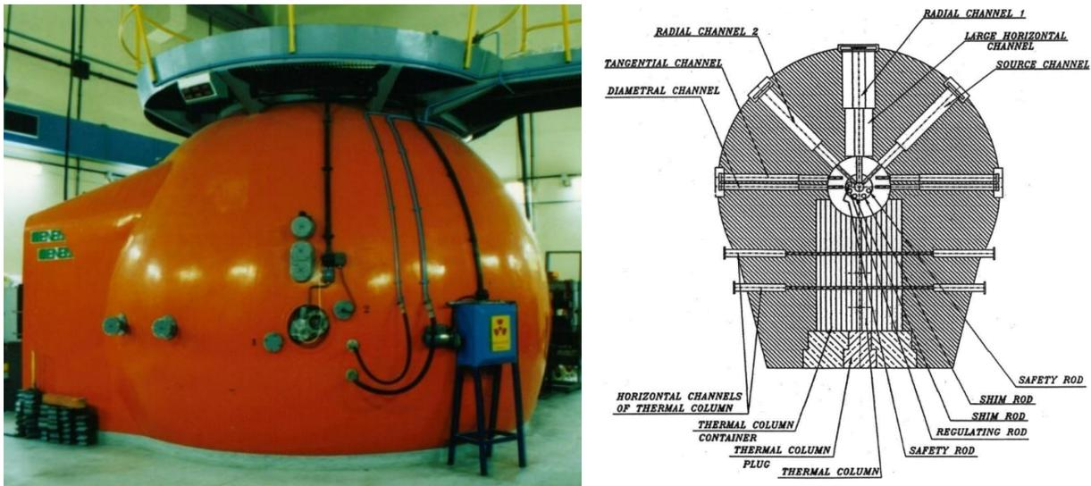
Figure 1. The TAPIRO research reactor (left) and its horizontal centre core cross section (right).
