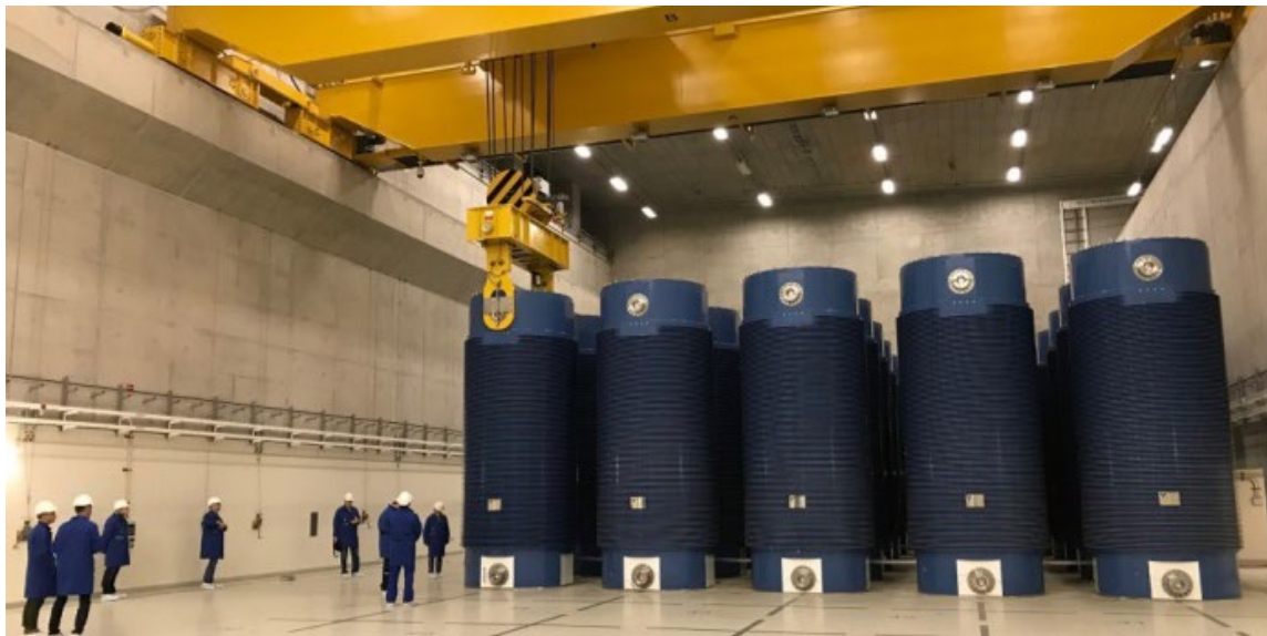
Figure 2: Image of spent fuel casks at the SFSF Unterweser, Germany (source: bgz.de).
