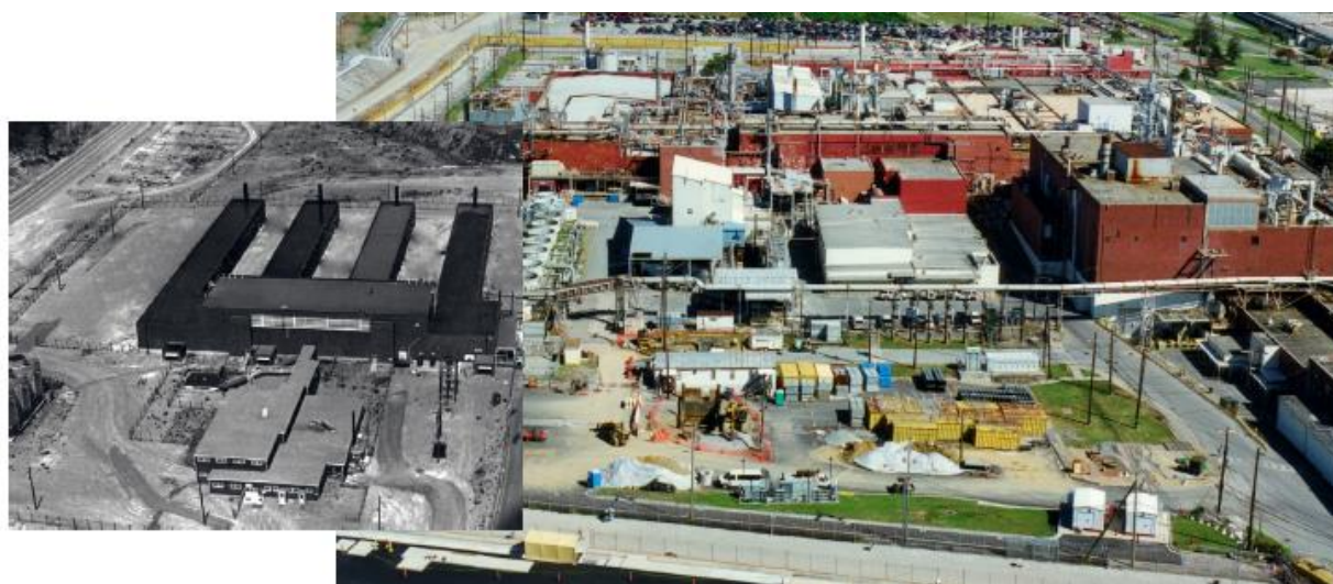
Figure 2. Building 9212, after construction (left) and the current Complex (right)
