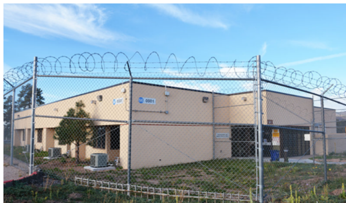
Figure 1-Safeguards Training Facility Located at TA-66.
