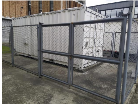
Figure n.º 2: Container for provisional storage of radioactive sources.
