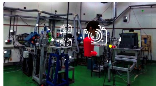
Two JRC cyclotron beam lines and target facilities
